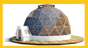
A geodesic dome is a partially spherical structure made of a network of triangles or combination of hexagons and pentagons. The geometric arrangement of these shapes help form a strong and structural support by evenly distributing its weight across the structure. Because of this, fewer materials can be used while maintaining the same strength as the traditional domes or buildings. The geodesic dome was also introduced as an energy efficient model.
